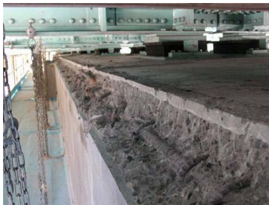
Fig. 2 Chipping inspection of pier beam.
