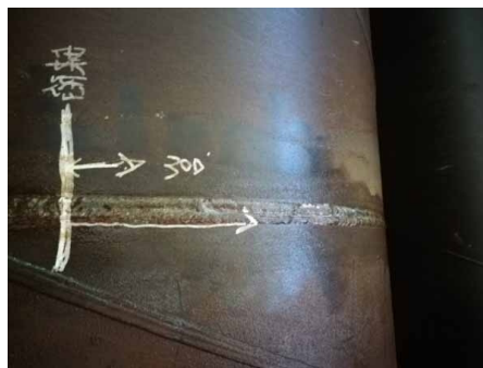
Figure 12. Failure modes of the test pipe [44].
