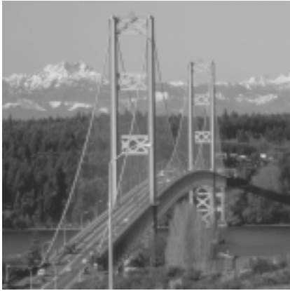
Figure 7. Original bridge image
