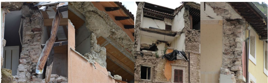
Fig. 4 Damage of different structural elements of the neighboring masonry buildings located in the historical centre of Visso, useful 178 also to understand structural details of the case study
