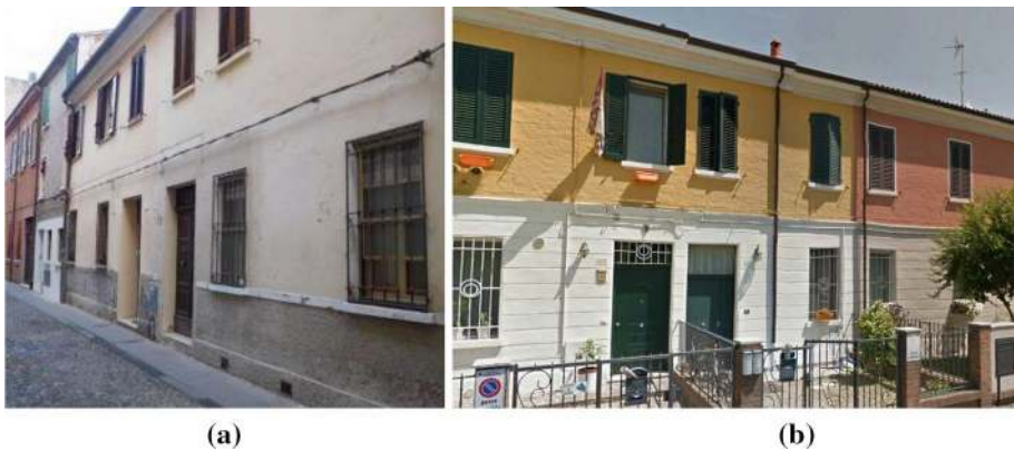
Fig. 3 Example of buildings MUR 2 class
