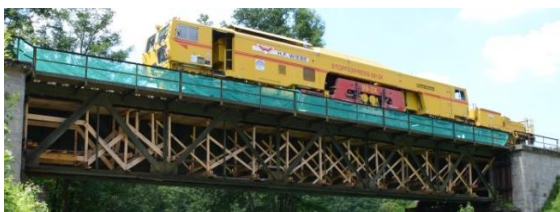
a) Track construction machinery on bridge
