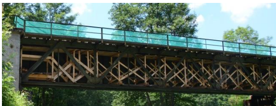
a) Photo of the bridge
