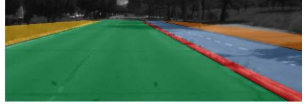
(a) The scene is composed (from left to right) by trees, 6.5 meters wide road, curb, bicycle way, small curb and sidewalk
