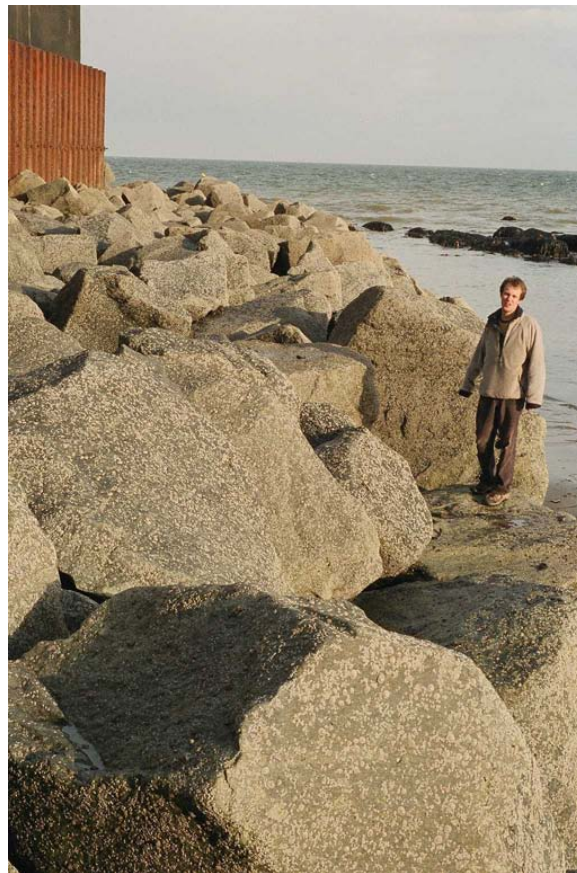
Figure 9: Samphire Hoe: Exposed rock toe at low tide (Courtesy of T Pullen, HR-Wallingford)
