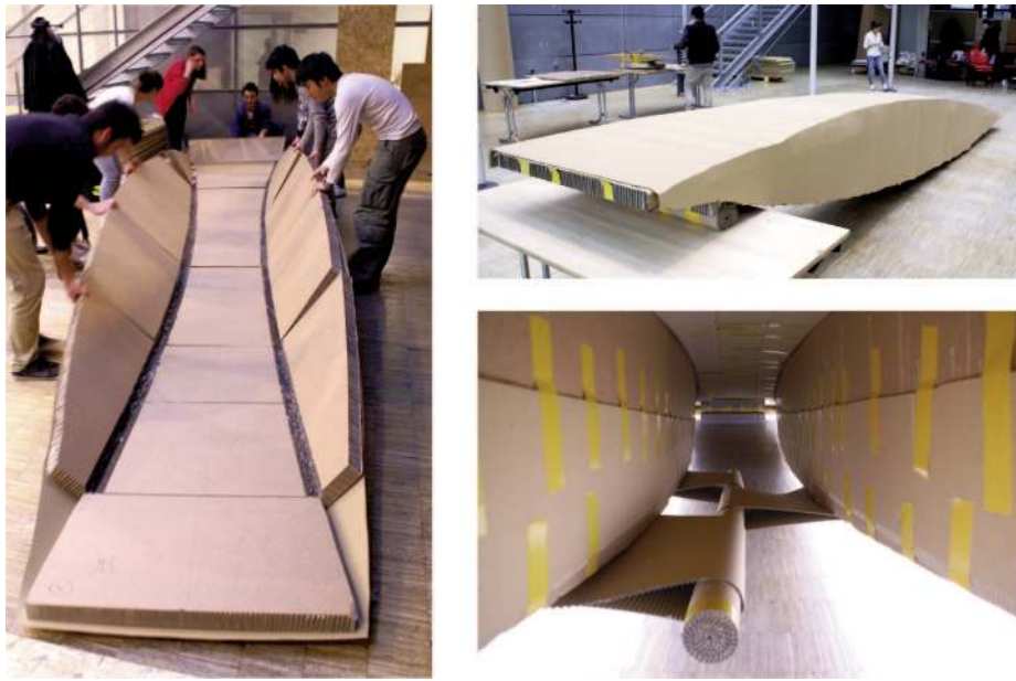
Figure 32. A foldable bridge made of corrugated cardboard and cardboard honeycomb. (Teachers: A. Lebée, M. Bernard, C. Chalumeaux, P. Lecomte; Students: M. Heinrich, N. Berrebbi, M. Kowalewski, A. Gauthier, S. L. Lee, J. Zagury, L. Gustin, L. Chassin, T. Biancone, R. Lévy).
