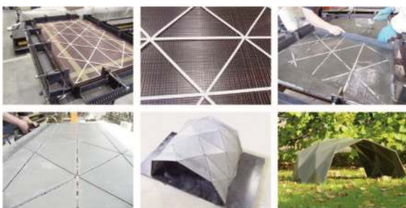
Figure 21. The fabrication and erection steps of a small scale oricrete [115].
