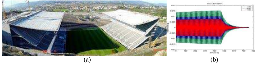
Figure 19. (a) Braga stadium's cable roof; (b) Measurement of modal free vibration response at three different points of the cable-roof after inducing resonance.
