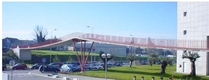
Figure 21. Stress-ribbon footbridge at FEUP Campus.
