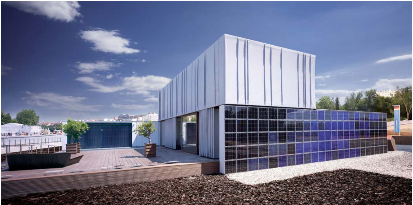
FIGURE 2. The building entered by Wuppertal University in the Solar Decathlon Madrid, 2010. The energy supply is based on solar power generation and vacuum tube collectors combined with a heat pump. Photo: Peter Keil, Düsseldorf.
