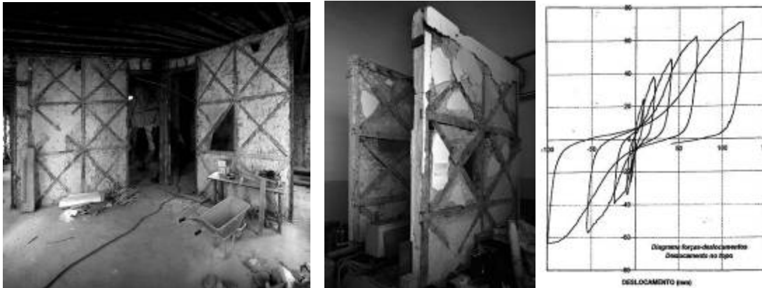
Figure 12: (a) 18th Century building in central Lisbon showing “Pombalino gaiola ” construction, 2003. (b) Gaiola wall sections from a late 18th or early 19th C. building after having been tested. (c) Hysteresis diagram from one of the wall tests of the walls in figure 12b.
