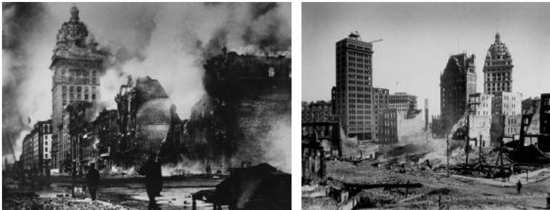
Figure 13: (a) Market Street, San Francisco during the post-earthquake fire of 1906, showing how even the new skyscraper of fireproof construction, the Hearst Building, caught fire from the wood windows and interior finishes (Bancroft Library). This building is still extant in 2006 in a remodeled state.
