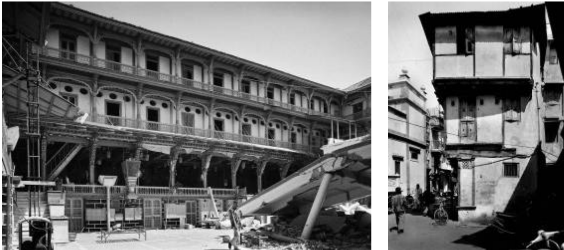
Figure 10: (a) Undamaged timber-laced masonry Swaminarayan Temple in Bhuj after earthquake. (b) Timber-laced masonry building in Ahmedabad historic walled city area after earthquake.
