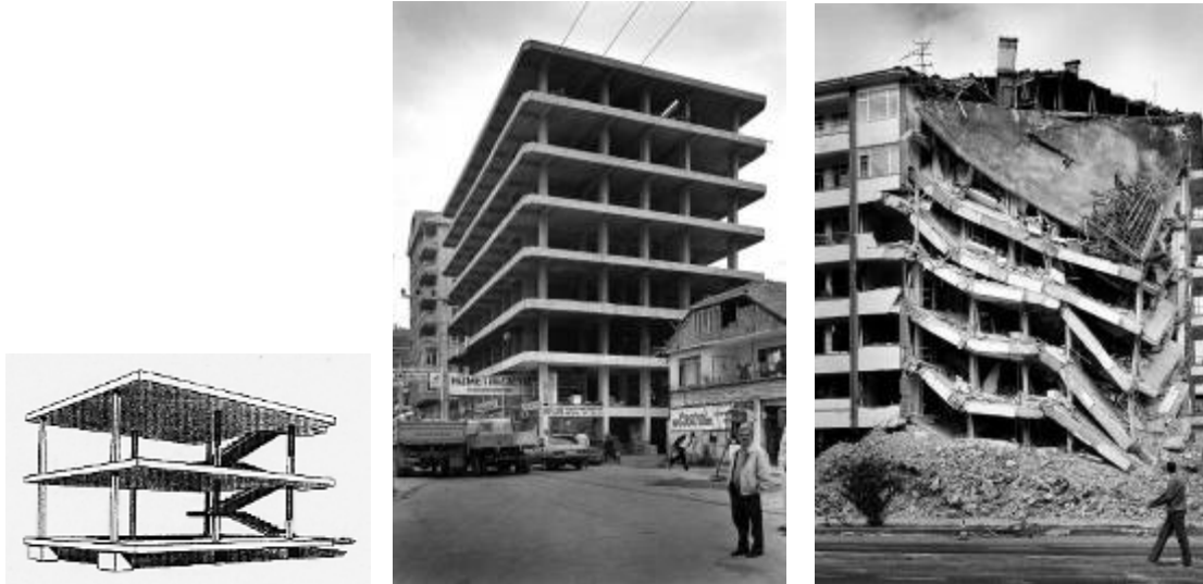
Figure 15: (a) Le Corbusier's conceptual Dom-Ino House, 1915 (b) Building under construction in Gölcük at time of 1999 earthquake (c) Partially collapsed reinforced concrete infill-frame building in Gölcük, 1999.
