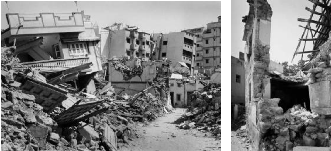
Figure 9: (a) Walled city area of Bhuj after 2001 earthquake. (b) Top-heavy thick masonry walls with shallow joist pockets collapsed easily.
