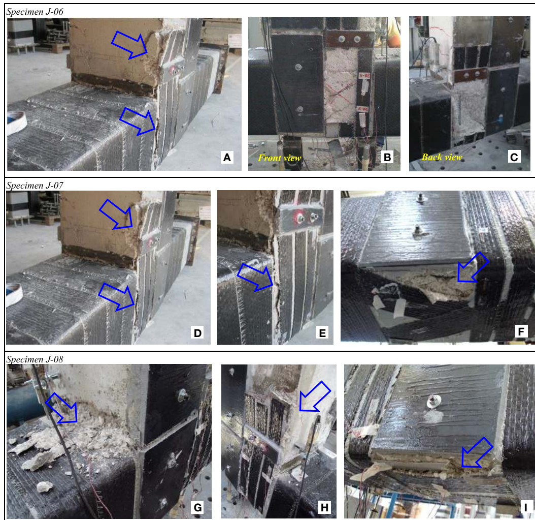
FIGURE 7 | Crack pattern and failure for CFRP strengthened specimens: J-06 (A-C); J-07 (D-F); J-08 (G-I).
