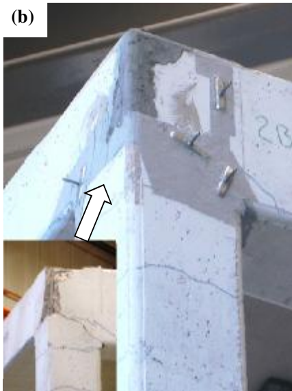
Fig. 9. Repairs after Phase 1: (a) welding of external beam bars to column bars, (b) mortar repair at J2B-2 and injection ports for crack injection, (c) crack injection in progress
