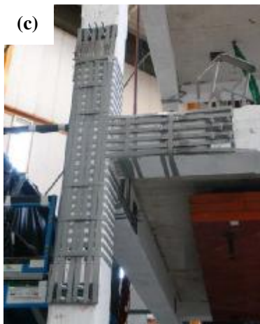
Fig. 11. PTMS strengthening of beam-column joints: (a) fixing of steel plates, (b) additional anchorage plate at interior face of beams, (c) final view of 1 st floor joints, (d) final view of 2 nd floor joints.
