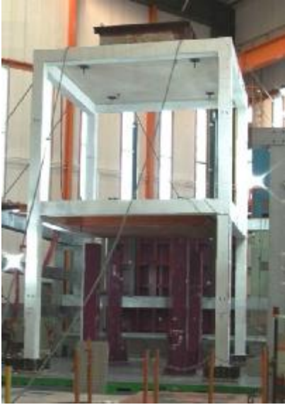
Fig. 2. General view of BANDIT building in bare condition
