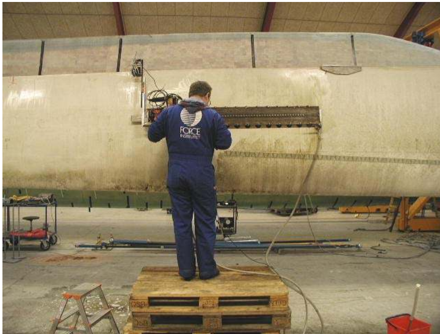
Figure 41. The flexible scanner mounted by means of vacuum on the wind turbine blade (damage no. 1).
