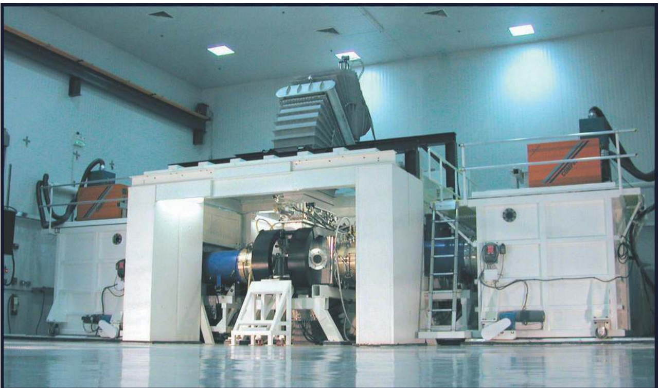
Figure 6. The Electra Laser Facility. Electra has repetitively produced 500 J per pulse of laser light.
