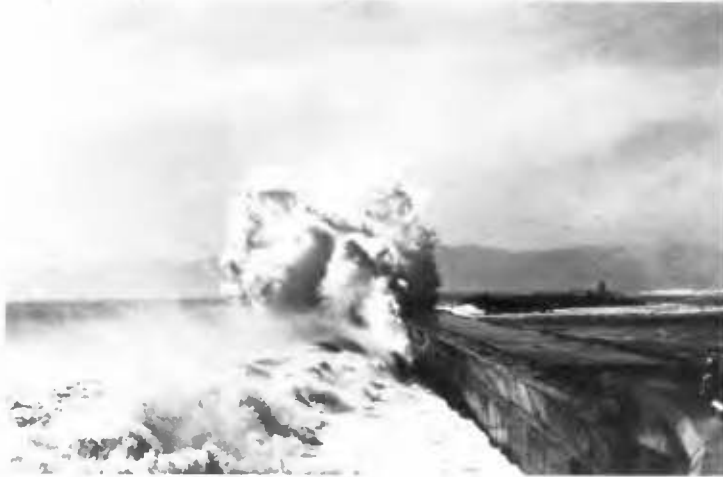
Fig 5. Wave attack on vertical breakwater
