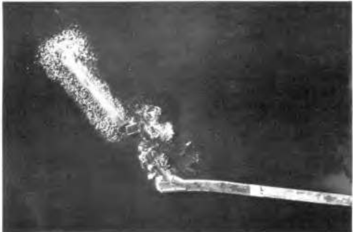
Fig 10. Storm damage to rubble mound breakwater
