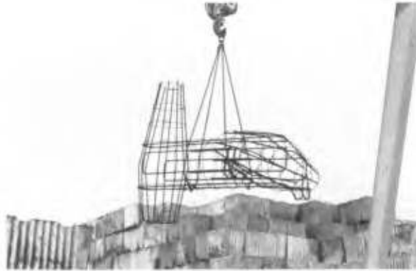
Fig 9. Reinforcing of toe dolos
