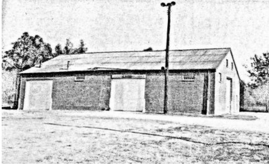
One of many of the Motor Vehicle Storage Buildings (MVSs) built in Louisiana post-WWII that also commonly served as armories (courtesy of LANG Archives).
