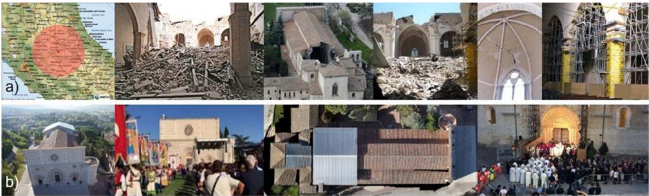
Fig. 1 Photographic sequence showing (a) the area stricken by the 6th April 2009 earthquake and the damages occurred to the Basilica and (b) the provisional covering realized after the seismic event and the opening of the Holy Door during the Jubilee Forgiveness procession
