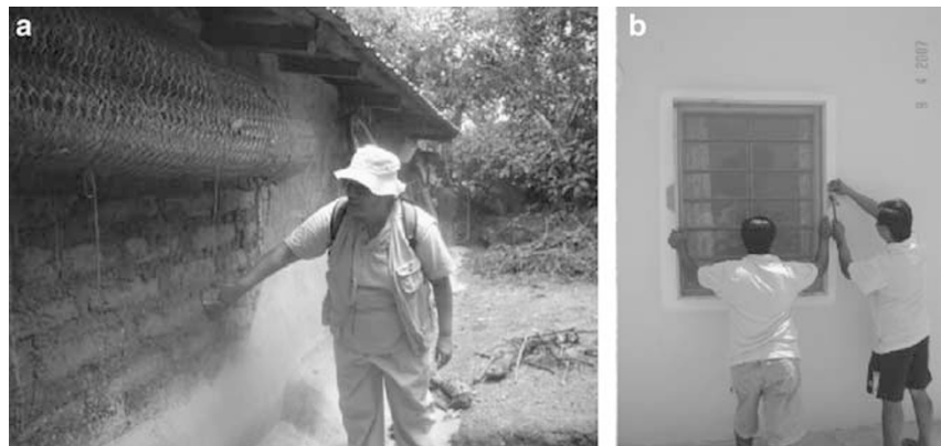
Figure 4 Innovative vector control interventions. Novel interventions, based on detailed knowledge of triatomine species population dynamics and genetics, may rely on improving wall plastering of houses using traditional methods, which prevents colonization (a), or on the installation of insect screens on windows, to prevent transient infestation (b).
