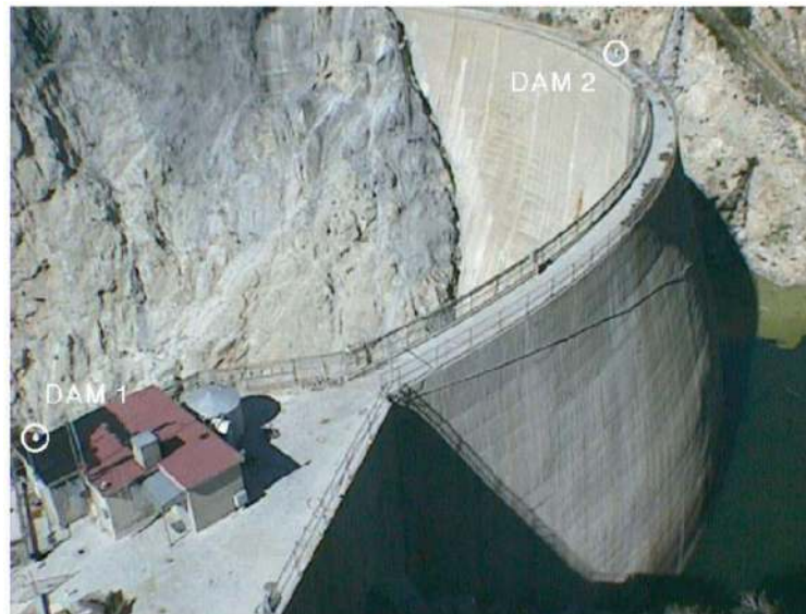
Figure 2. Example of the GNSS (Global Navigation Satellite System) continuous recording stations DAM1 (reference) and DAM2 (CP) at Pacoima dam, USA (image credit: J.A Behr, 1998, https://pasadena.wr.usgs.gov/office/hudnut/SRL/figures/Figure_1.gif ).
