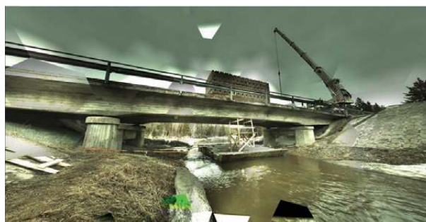
Fig. 4. Full load (1961 kN) placed on the bridge, image view from the scanners position from the Southern side of the bridge
