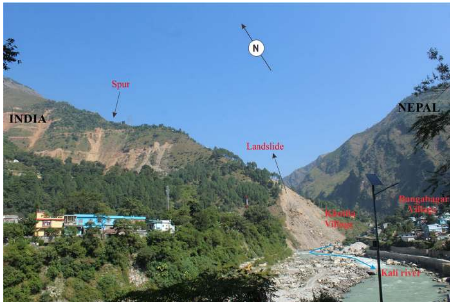
Figure 4. Panoramic view of the Khotila landslide.
