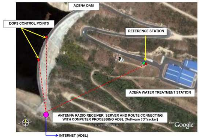
Fig. 6 DGPS spatial arrangement in La Aceña Dam
