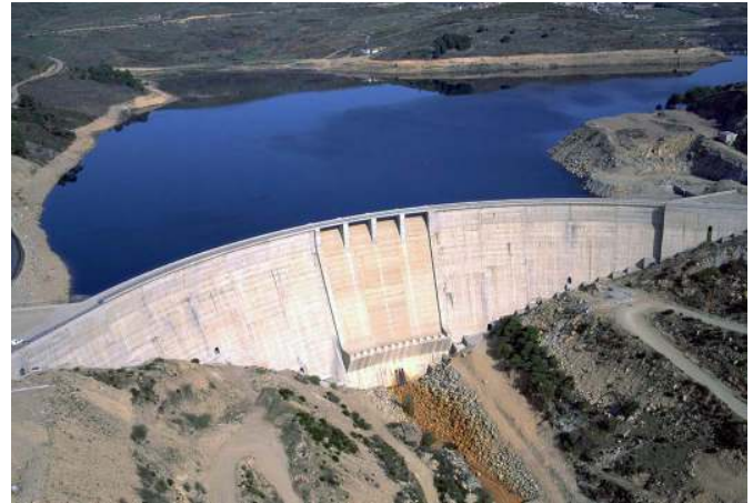
Fig. 1 La Aceña dam (Central Spain). General view
