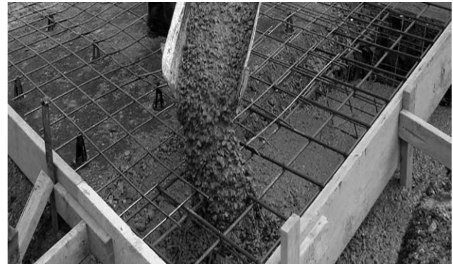
Fig. Geopolymer Concrete in Reinforcement
