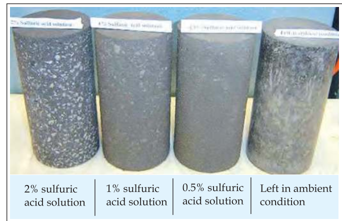
Figure 6. Visual Appearance of Heat-cured Geopolymer Concrete after One Year of Exposure in Sulfuric Acid Solution [12]
