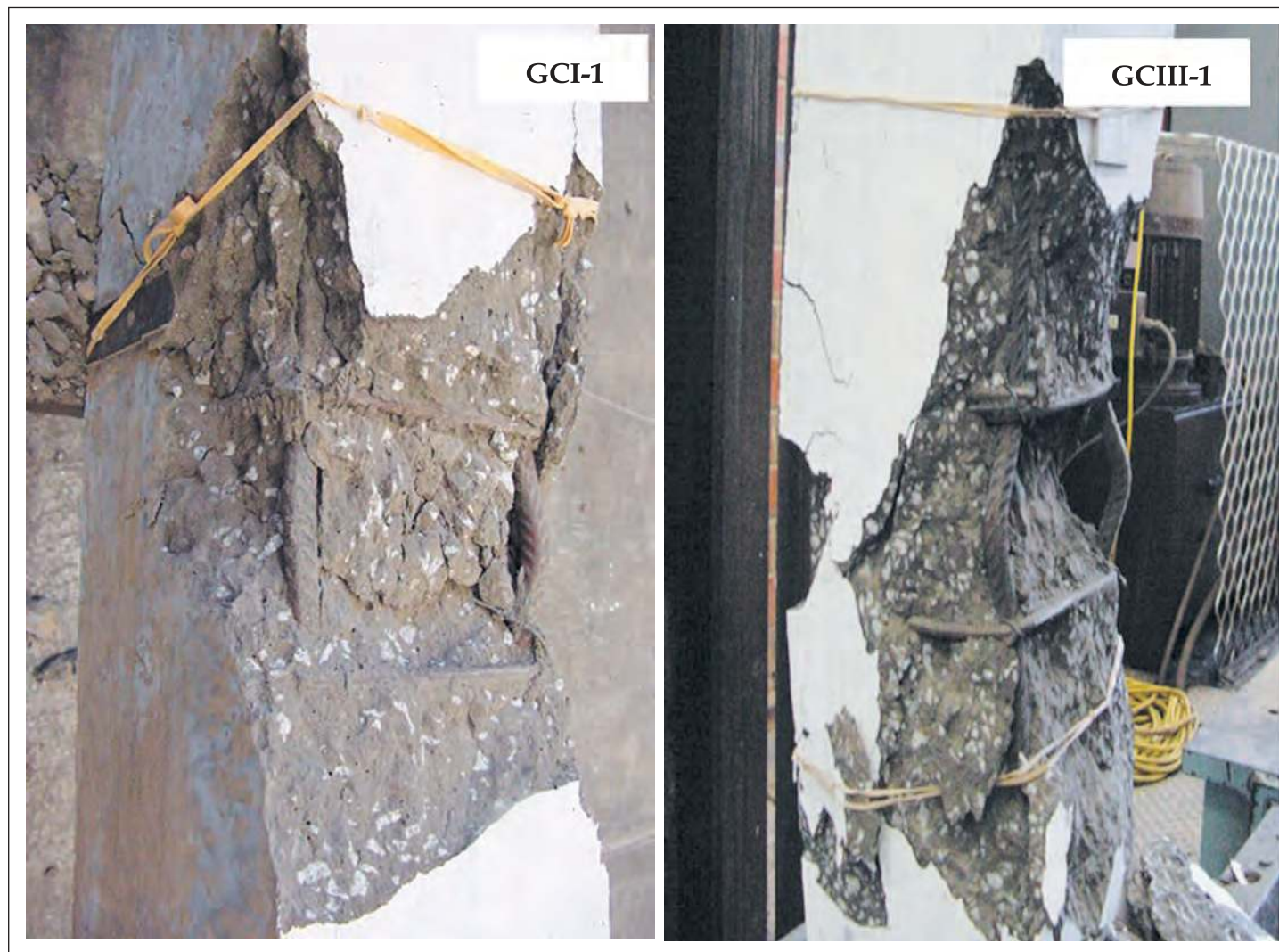
Figure 8. Failure Mode of Reinforced Geopolymer Concrete Columns [13]
