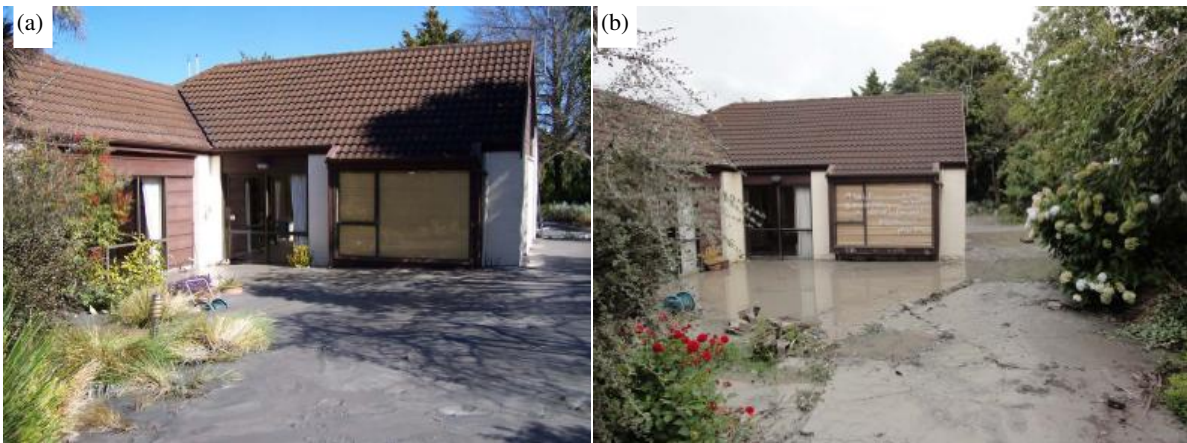
Figure 20: Illustration of a house in Kaiapoi which sustained liquefaction in both the (a) 4 th September 2010 Darfield; and (b) 22 February 2011 Christchurch earthquakes.
