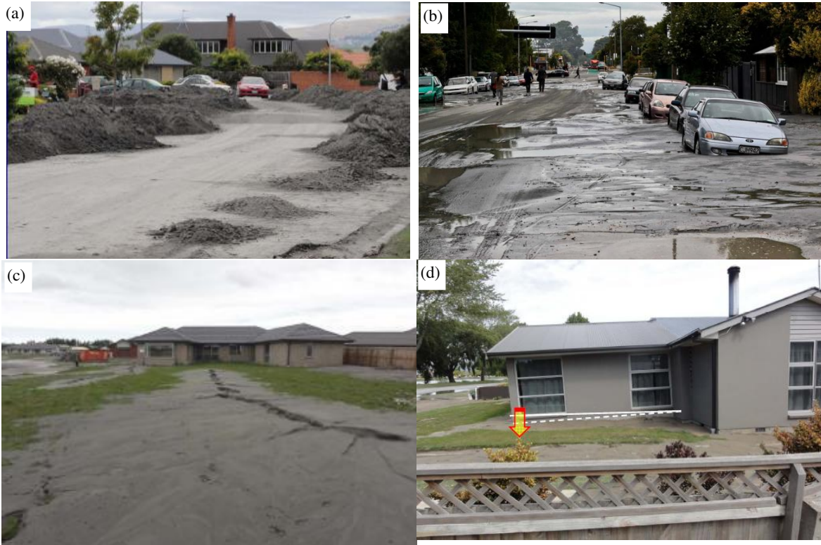
Figure 19: Typical manifestation of liquefaction in residential areas.
