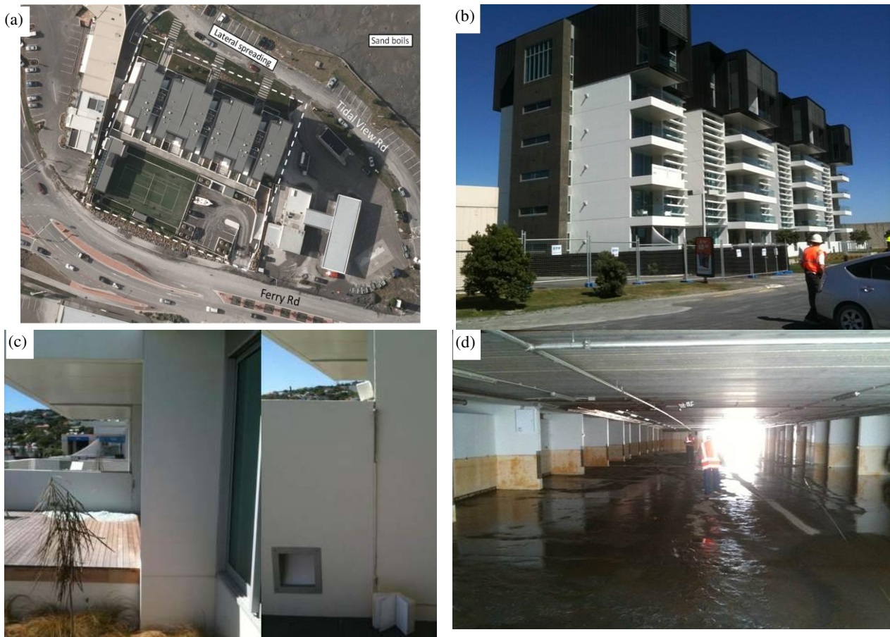
Figure 32: (a) Aerial view of Ferrymead apartment building indicating surrounding ejected material; and (b) south-west looking view of the apartments; (c) separation of walls on the north side of the building, including sloping of the separation walls and shattered glass panels, and compression of caulk at top of expansion joint; and (d) the basement parking garage. Note the high water mark on the walls.
