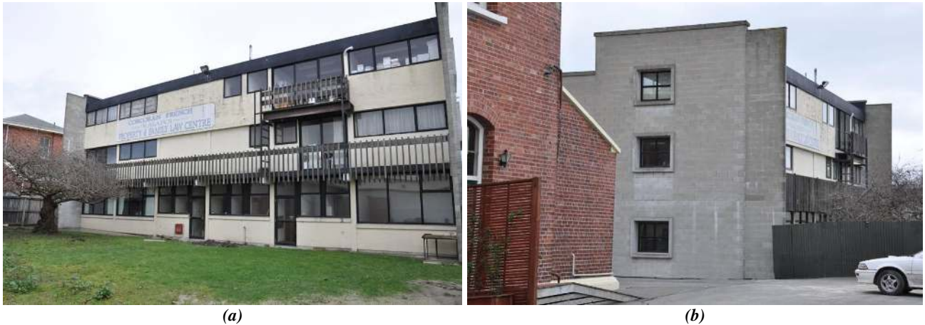
Figure 5.7: Property and Family Law Offices in Kaiapoi business district. (Williams St.) (a) View looking northwest (at long axis end) of building and (b) view looking northeast showing shear wall ends of short axis of building.
