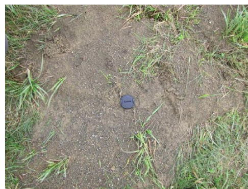
Figure 4.38: Liquefaction on the grass verge adjacent to the end of Gillanders Rd (Darfield side). Note the fine gravel particles on the surface and the fissure towards the top right hand side - it was possible to push the sampling spoon to a depth of about 300 mm into the fissure. (Position marked as Photo 2 in Fig. 4.36).
