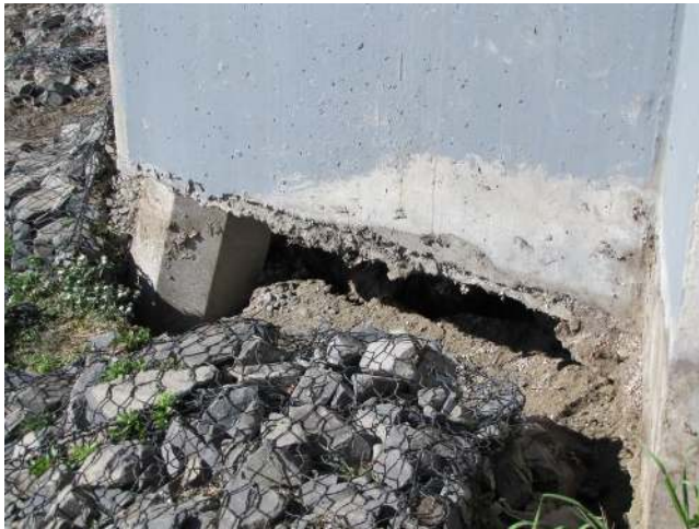
Figure 7.6: West abutment batter (angled) pile, Bridge Street Bridge.
