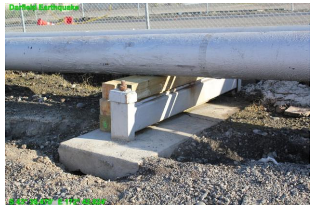
Figure 7.38: Temporary wooden support to accommodate settlement under fuel line.
