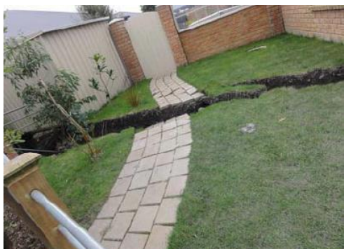
(a) Large ground cracks due to lateral spreading at Kokopu PI; (d) Cracks in unreinforced slab induced by lateral spreading.
