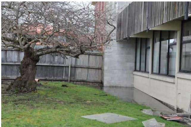
Figure 5.8: Property and Family Law Offices in Kaiapoi business district. (Williams St). View looking at west short axis end of the building.
