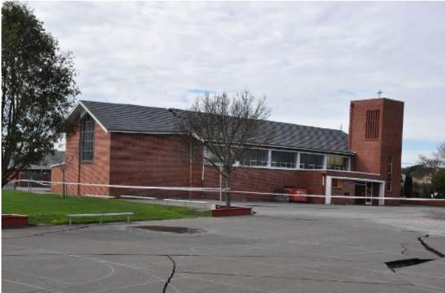
Figure 5.30: St. Paul's church in Dallington area - overall view of building looking north-east.
