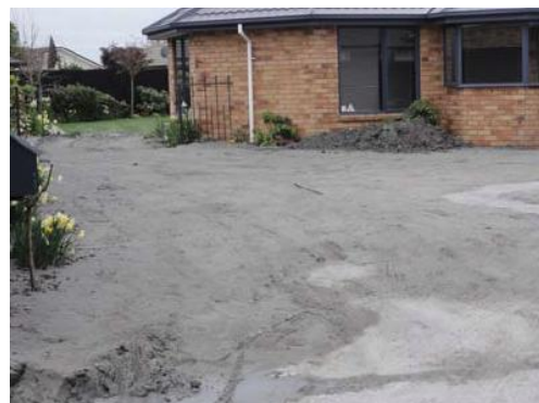
(a) Aerial view of the southern edge of Bexley which was severely affected by liquefaction and lateral spreading; (b) Evidence of liquefaction in residential area (Seabreeze CI).
