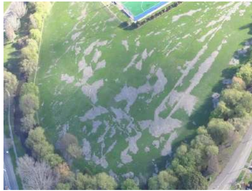
(a) Aerial view: massive sand boils with large number of parallel cracks along drainage lines (from a helicopter flyover on the afternoon of Friday September 10).
