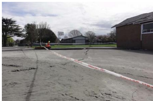
(b) Evidence of liquefaction in foundation soils resulting in large total and differential settlements.
