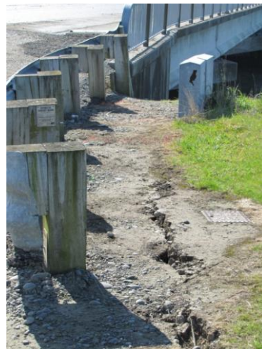
Figure 7.2: Cracking on margins of west approach embankment, Bridge Street Bridge.
