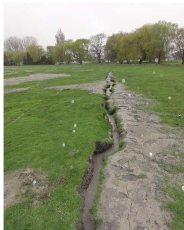
(b) ~10 cm wide lateral spread crack.
