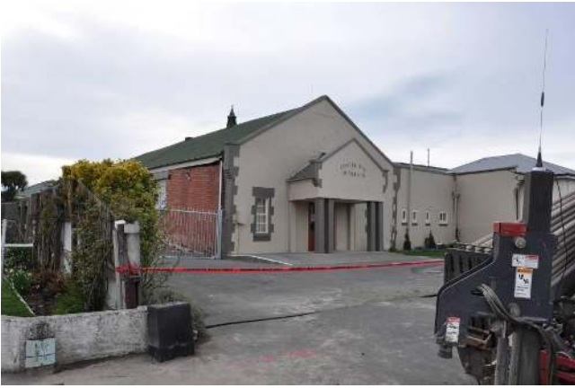
Figure 5.3: Front facing (view looking northeast) of the Gospel Way church in Kaiapoi along Charles Street.
