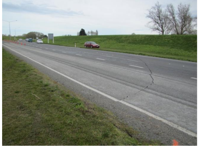
Figure 7.26: Cracking in and along roadway adjacent to Chaney's Overpass.
