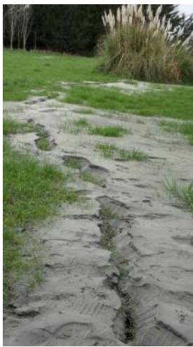
Figure 6.28: Liquefaction and lateral spread features on or near stopbanks located about 100 to 200 m west of the Kaiapoi Sewage Treatment Plant. (upper left: 43.389175°S, 172.683235°E; upper right: 43.389701°S, 172.683390°E; bottom left: 43.389519°S, 172.682203°E; bottom right: 43.389432°S, 172.6682060°E).
