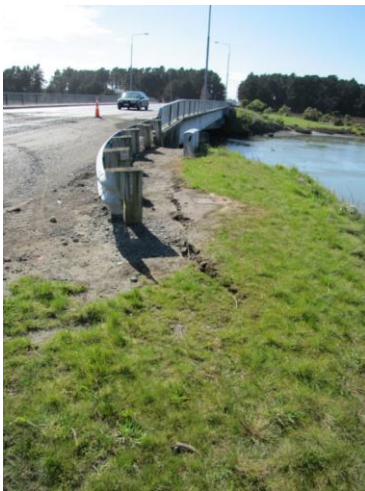
Figure 7.2: Cracking on margins of west approach embankment, Bridge Street Bridge.
