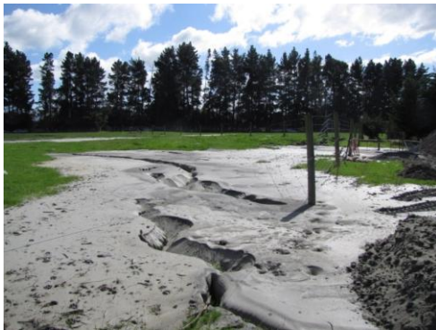
Figure 4.32: Sand boils in fields (position 2; 43.4026°S, 172.6503°E).
