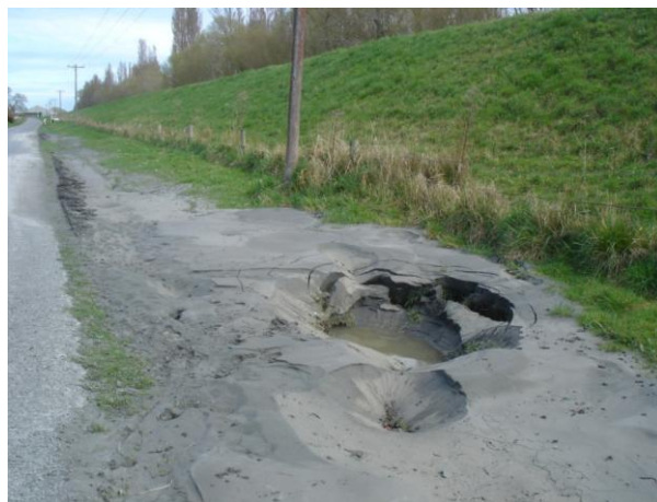
Figure 6.4: Photo 1: Large sand boil at the base of the landside of the stopbank on Coutts Island Rd. (43.425018°S, 172.628442°E).
