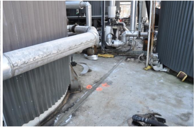
Figure 7.44: Repair of lateral spread cracks within the Fulton Hogan Bitumen Plant, nearby Tank 3. (43.6085°S, 172.7150°E).
