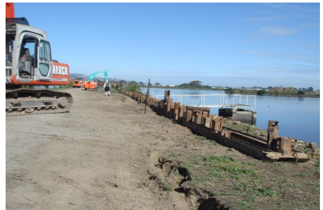
Figure 6.34: Sheetpiles being driven to stabilize the pond embankment to arrest further movement. (-43.530563°, 172.718349°).
