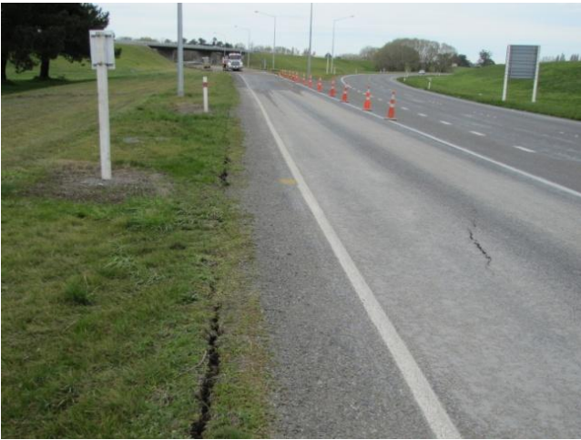
Figure 7.26: Cracking in and along roadway adjacent to Chaney's Overpass.
