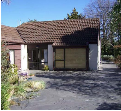
(a) ~400 mm thick layer of silt-sand-water mixture covering a residential property affected by very severe liquefaction; (b) same-angle view, but after the clean up of sand boils.
