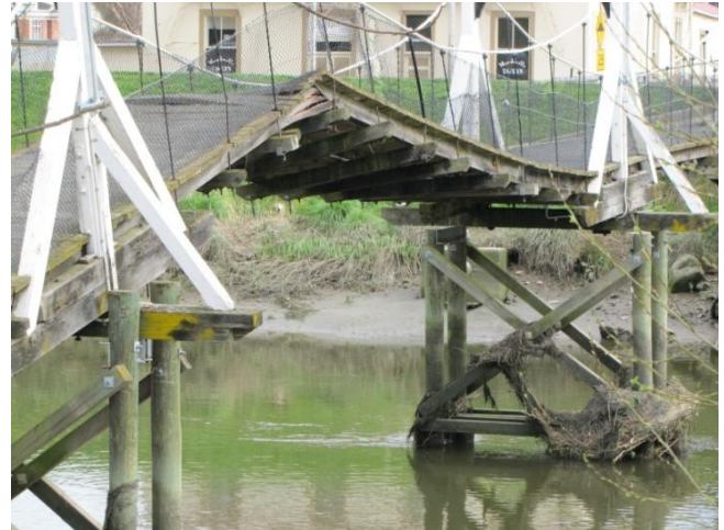
Figure 7.19: Buckling of footbridge near Trousselot Park.
