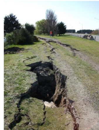
Figure 6.33: Lateral spread cracks at the eastern end of Pond 2B. The sink hole in the foreground of the photo on the right formed over the top of two outlet pipelines. (-43.52895°, 172.717300°).
