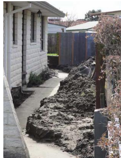
(a) Evidence of extensive liquefaction at the east end of Charles St.
