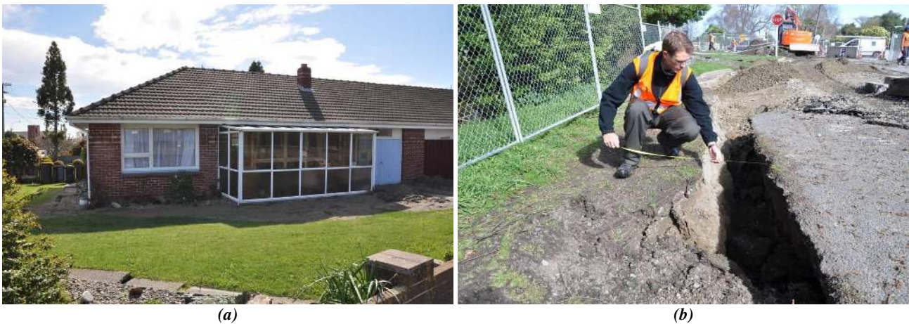
Figure 5.25: (a) Rigid body rotation of a residence in Dallington (Locksley Avenue) due to liquefaction and (b) lateral spread features directly fronting the home. Surveys of ground features at this location are associated with T7 (refer to Figure 5.27).
