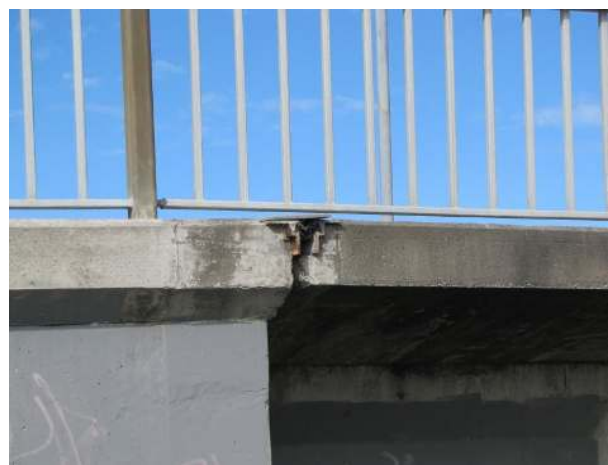
(b) East abutment gap closure.
