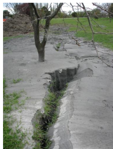
Figure 6.19: Photos 19-20: Lateral spreading cracks along the landside of the stopbank on the north side of the Kaiapoi River. The locations of these photographs are denoted in Figure 6.2. (43.384633°S, 172.661231°E).
