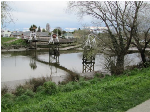
Figure 7.19: Buckling of footbridge near Trousselot Park.
