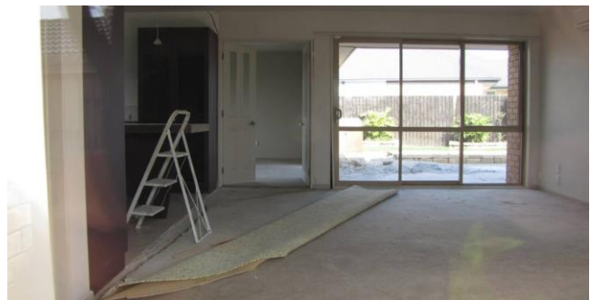
Figure 5.39: Fissure in concrete floor slab (to the left hand side passing beneath the ladder). (Same house as in Figure 5.38.) (Kokopu Street).
