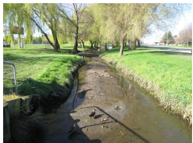
Figure 4.20: Photograph of the stream near Porritt Park on Wednesday, 15 September 2010. There is lateral spreading towards this stream from both sides. It is just possible to make out a sand boil in the midst of the stream bed debris to the right of the duck. Several other sand boils were visible along the stretch of heaved stream bed.
