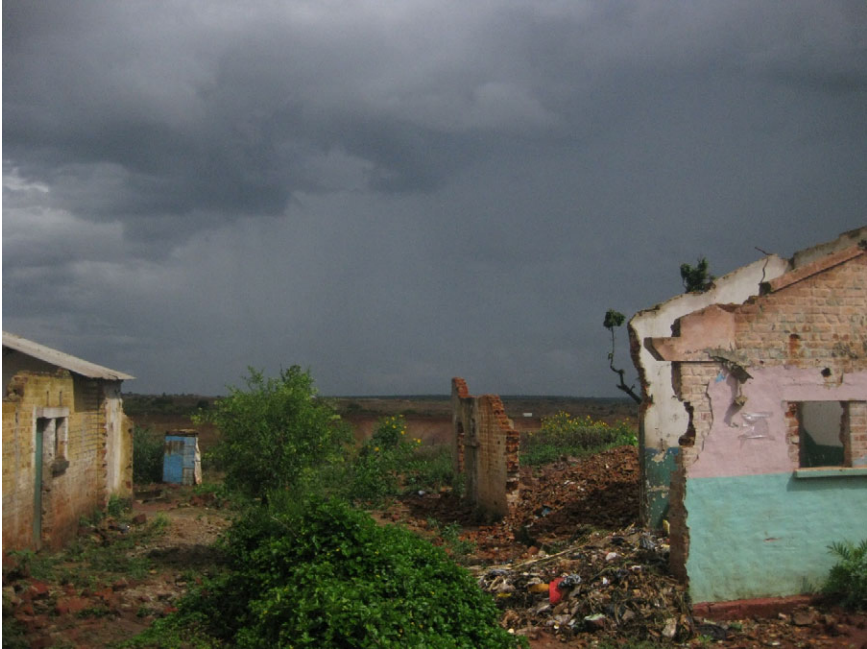
Figure 5. Ruins of the houses in cité Gécamines that were abandoned to make room for the mining activities as the open pit in the background expanded. Source: the author.
