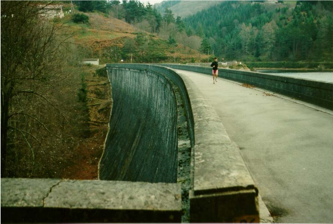
(a) View of the downstream dam face from the left bank.
