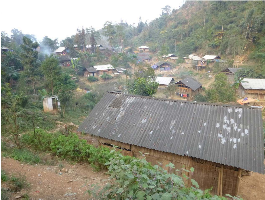
Photo 6.2: A poorer village in the commune. Note the houses with new asbestos roofing, provided as part of the government's poverty reduction support
