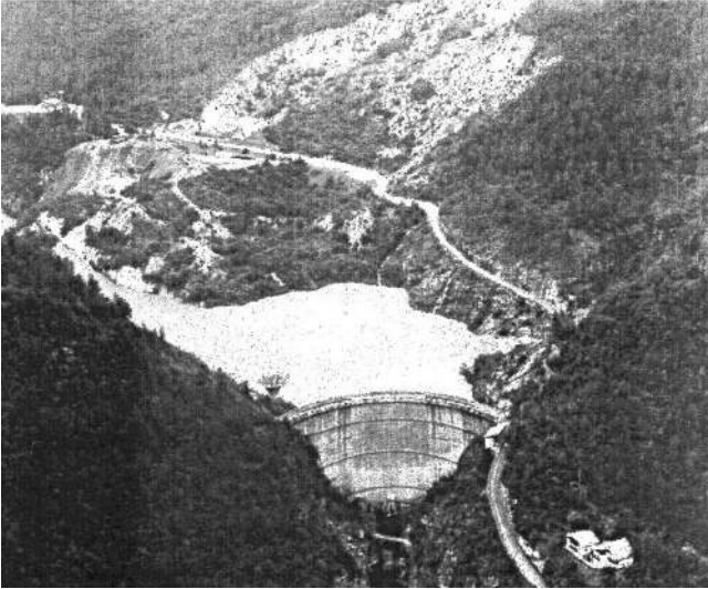
Fig. 5. Picture of the Pontesei dam and artificial reservoir as it appears today. The 1959 landslide is clearly visible in the upper part of the picture.
