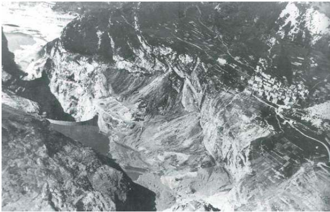
Fig. 12. The Vajont valley just after 9 October 1963, landslide event. In the left part of the picture it is possible to see the Vajont dam, as it is now, which was not damaged by the overtopping water.
