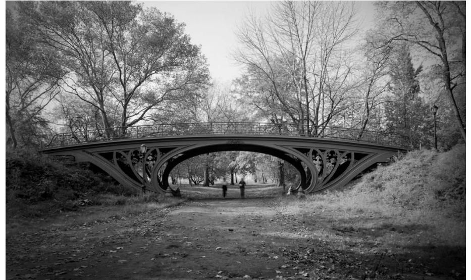
Figure 7. Gothic pedestrian bridge over bridle trail, Central Park. Source: Jet Lowe, 1984, Library of Congress; Historic American Engineering Record. Image in public domain.
