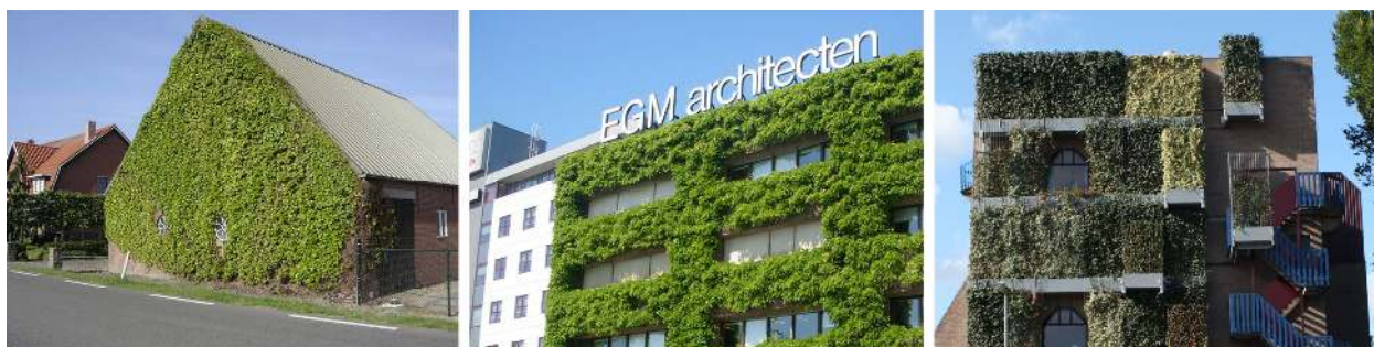
Figure 4. Direct greening system (a), indirect greening system (b), indirect greening system combined with planter boxes (c).
