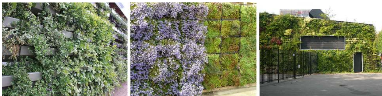
Figure 5. LWS based on planter boxes (d), LWS based on foam substrate (e), LWS based on felt layers (f).
