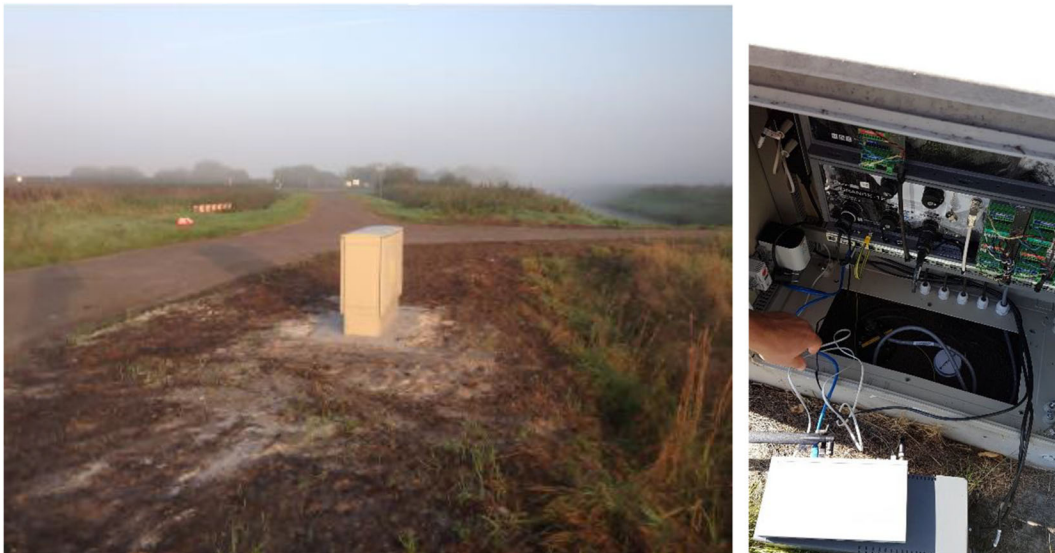
Fig. 6 Exterior (left) and interior (right) of a G-station. The stations were installed in remote locations to minimize the noise recorded
