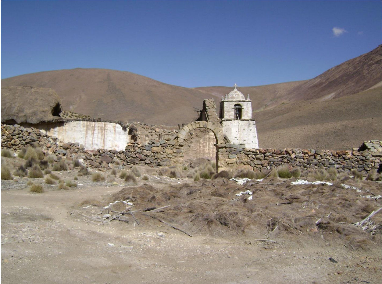
Figure 4.4 Church of Choquelimpe, with collapsed roof. Photo by the author (2009)
