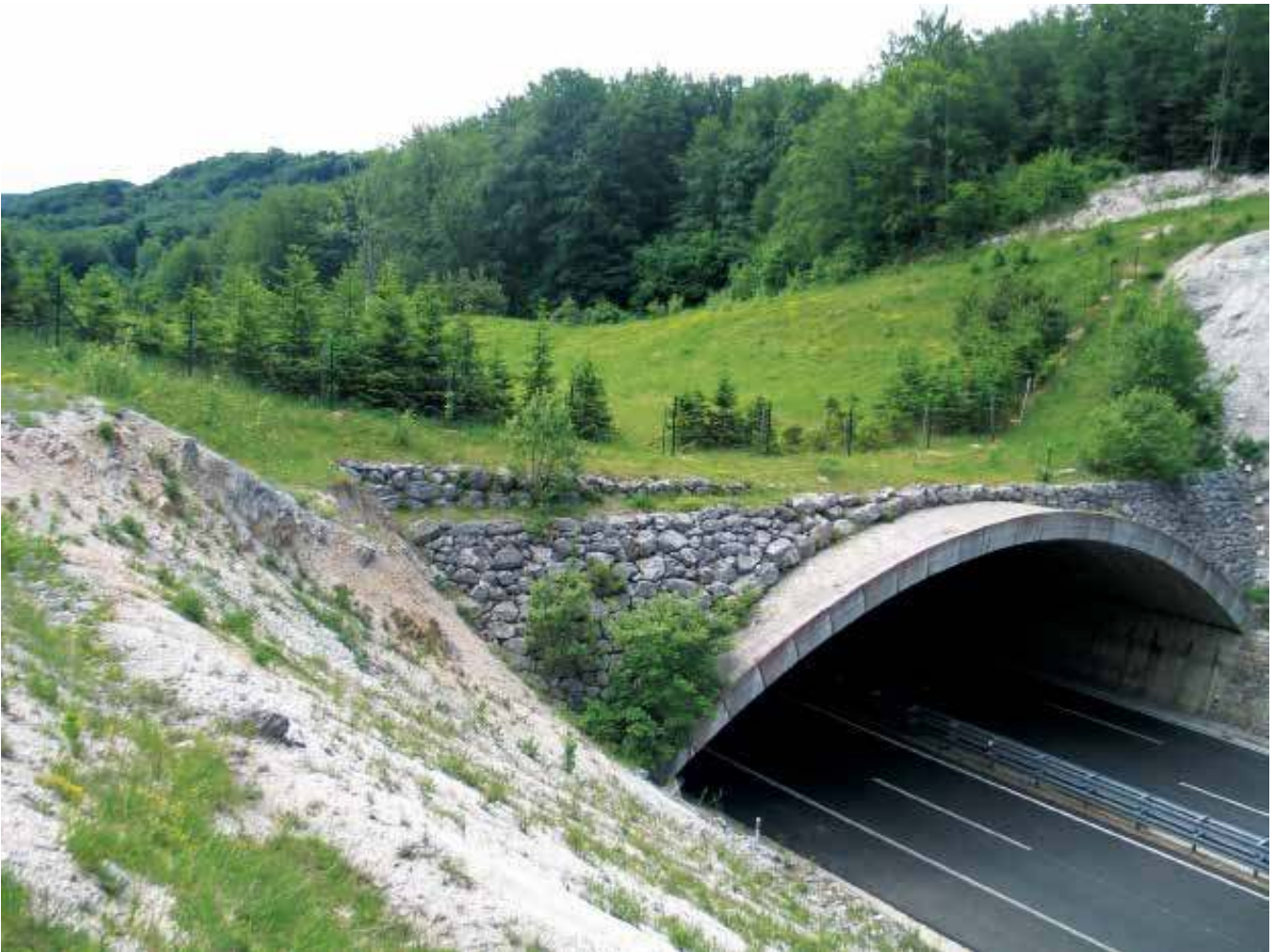
Wildlife crossing structures such as this highway overpass in Croatia, one of 13 in the country, are no substitute for an intact landscape but have value in mitigating the effects of fragmentation for many species. © Djuro Huber
