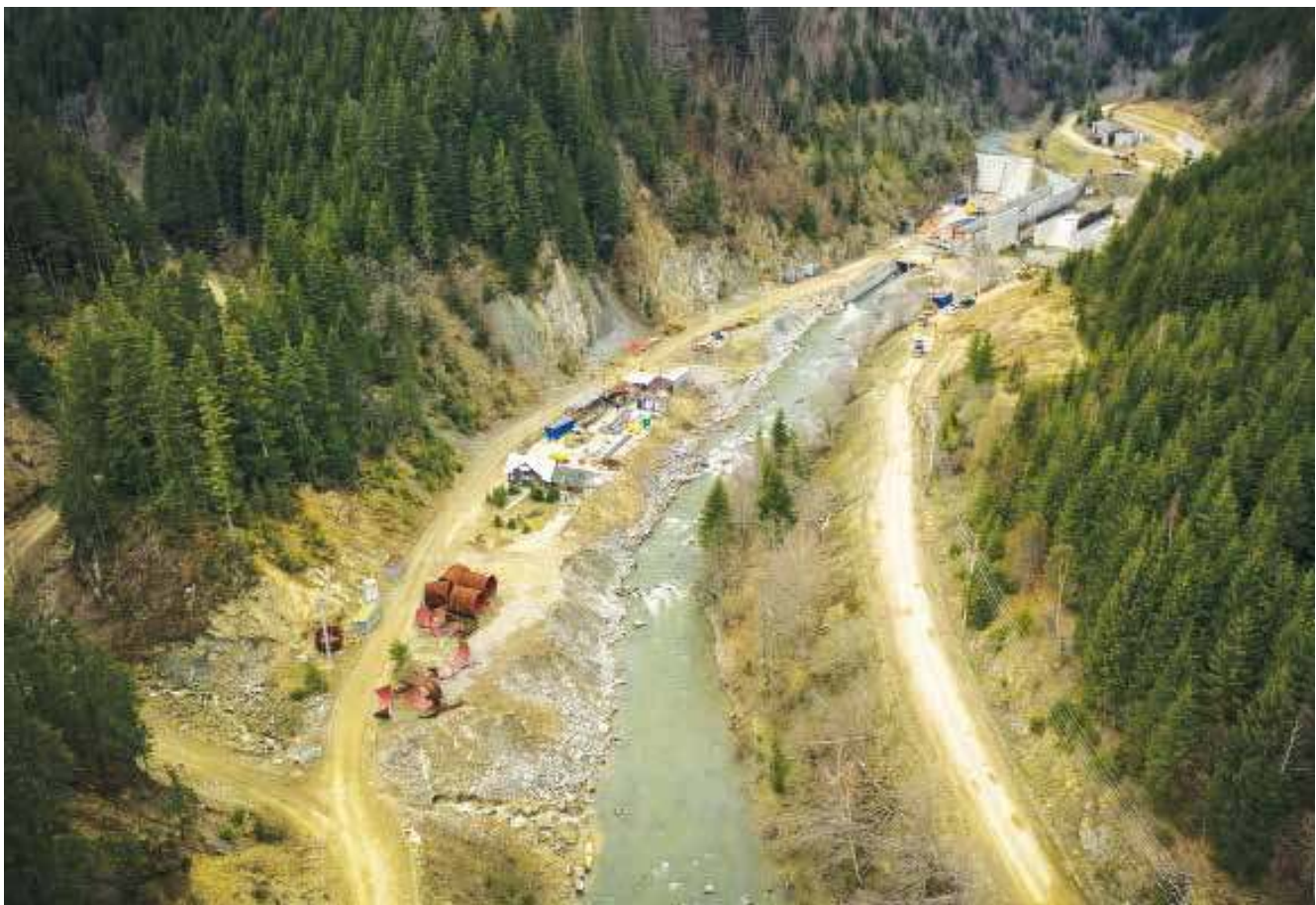
Just one third of the world's rivers remain free-flowing. Dams are the primary barrier to freshwater connectivity. Here, a dam is under construction on the emblematic river Bâsca Mare, Romania, found in the heart of the Carpathian ecoregion of Europe. © Leeway Collective / Balkan River Defence, Courtesy Calin Dejeu
