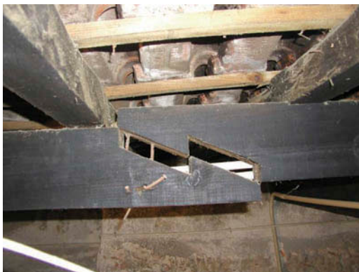
FIG. 12. Lack of contact and failure of the joint.
