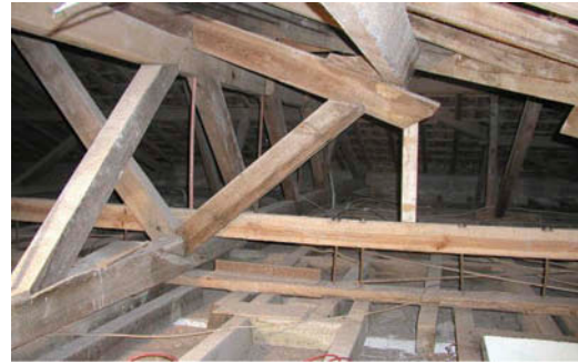
FIG. 7. Missing part of the structure due to previous interventions.
