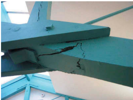
FIG. 6. Timber failure in the vicinity of the joint.
