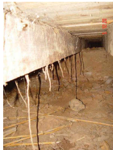
FIG. 9. Evidence of subterranean termites attack.
