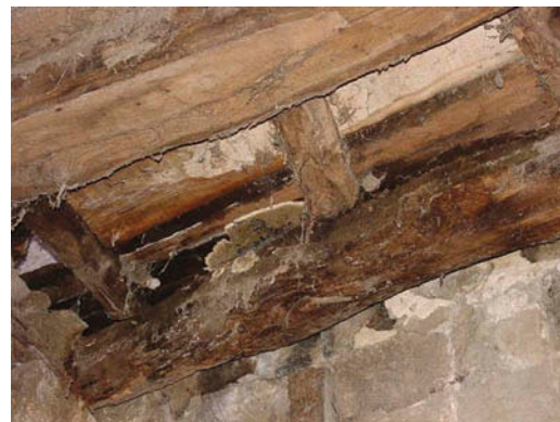
FIG. 10. Evidence of fungal attack.
