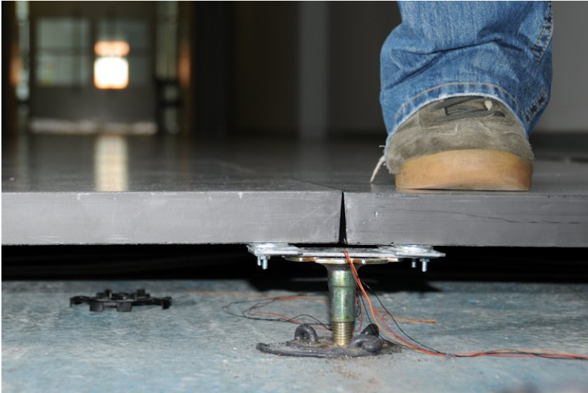
(b) Floor tiles rest on columns.
