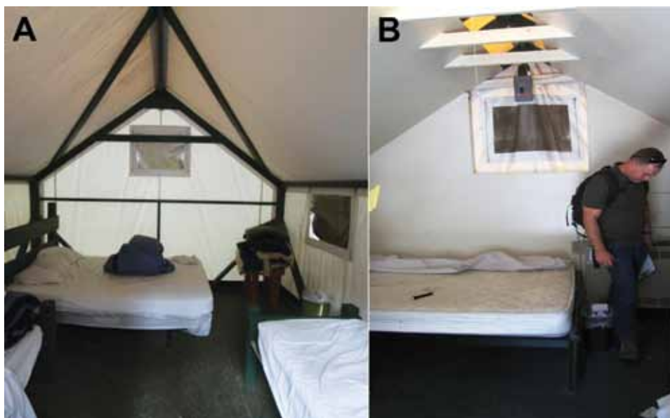
Figure 3. Inside view of regular and signature tent cabins, Yosemite National Park, summer 2012. A) Regular tent cabin showing canvas affixed over a wood frame. B) Signature tent cabin showing drywall between the exterior canvas and the interior living space.
