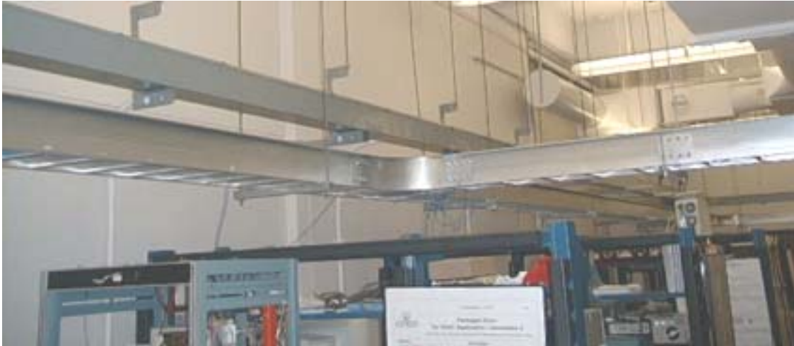
Figure 156: Photograph of cable tray system that forms the backbone of the laboratory-scale microgrid
