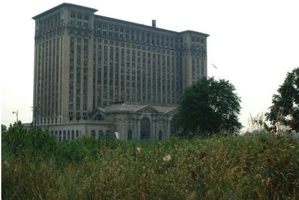
FIGURE 2. 'Ruin time': Detroit, abandoned train station with overgrowth. Photograph by the author, June 2005.
