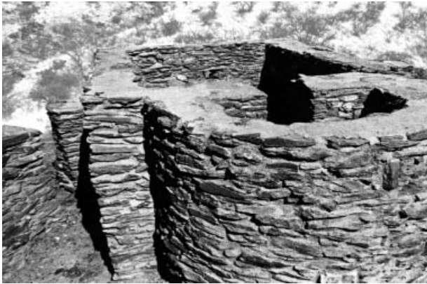
FIGURE 17. The Eros Fort outside Windhoek, built in 1893, present condition. Photograph courtesy of Dr Andreas Vogt, Windhoek/Namibia.
