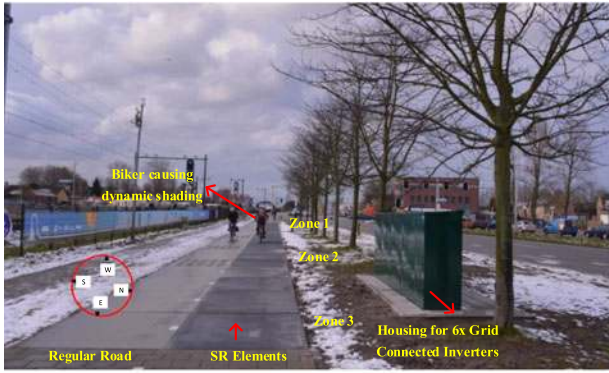
Fig. 1. Photo of the installed SR bike path. (For more information, see [25]).
