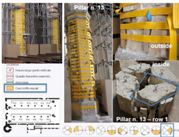
Figure 10. Pillar n. 13. A case of better ashlar stone conservation with respect to the hypothesized state of the art of the inner before disassembly and after reassembly. The external deterioration of the stone, in good condition in the inner part, is evident.
