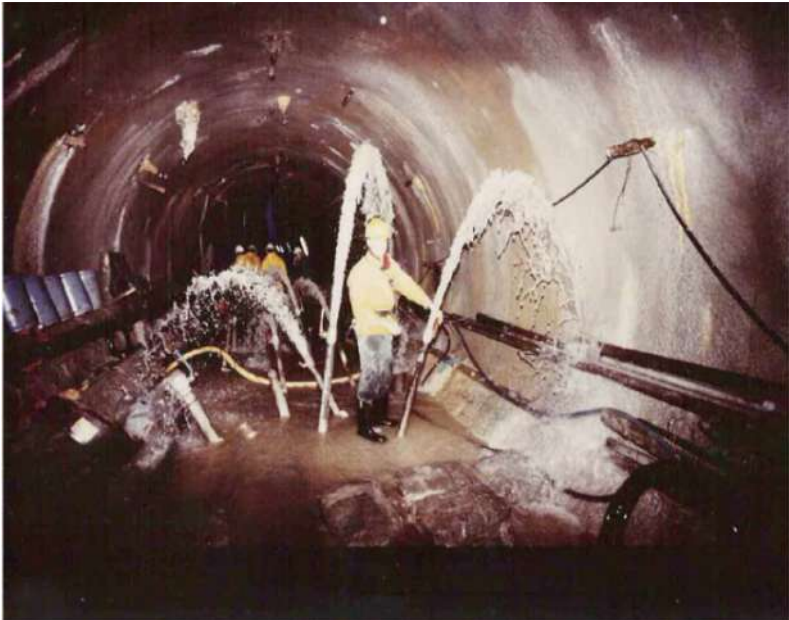
Fig. 4.10. Water inflows during LEP tunnel construction.
