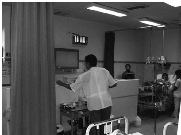
Fig. 17.6 Upper Room UV system (located on wall below ceiling) in a hospital ward. Image provided courtesy of Chuck Dunn, Lumalier, Memphis, TN
