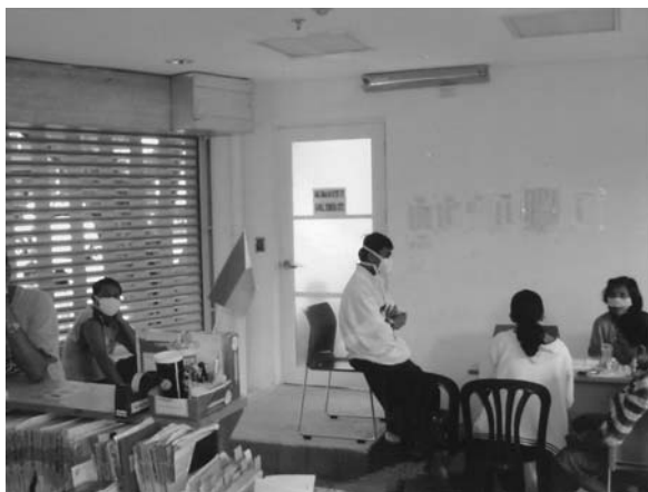
Fig. 17.10 Example of an Upper Room UV system (located at the ceiling) in a TB clinic. Photo provided courtesy of Pablo R. Antonio Designs and Consultancy, Inc. Makati City, Philippines
