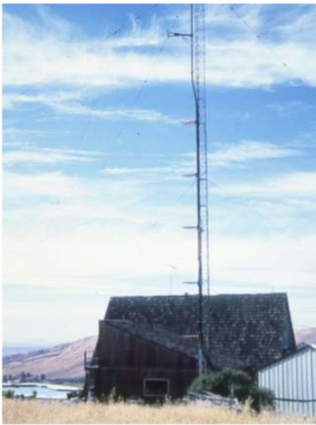
Fig. 15. House close to a radio broadcasting tower in San Jose - CA (photo by Richard A. Tell). The EMF field measured in the proximity of the house was higher than 61.4 [V/m].
