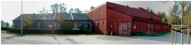
Figure 11. Main entrance (right) and residential units (left)
