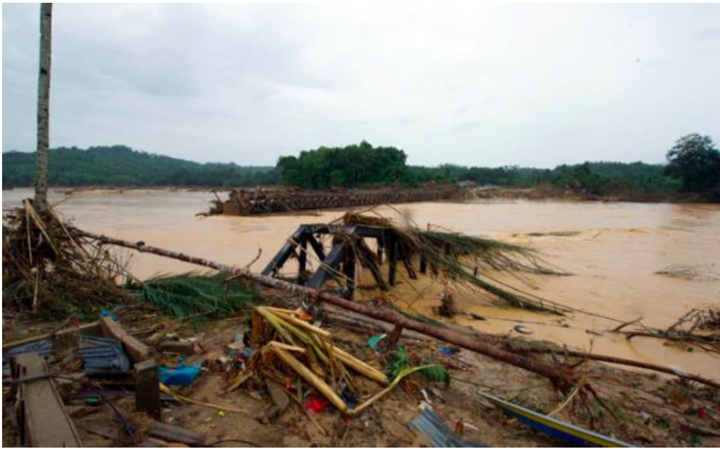
Figure 3: Malaysia East Coast Line railway bridge, which cross Nenggiri River in Kemubu, Kelantan had totally lost due to massive flood in December 2014. (Courtesy: SPAD)
