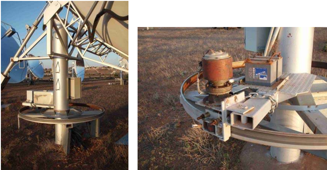
Figure 6-3. The “pipe-in-pipe” azimuth drives at White Cliffs required little maintenance during the 17-year operating history of the plant.
